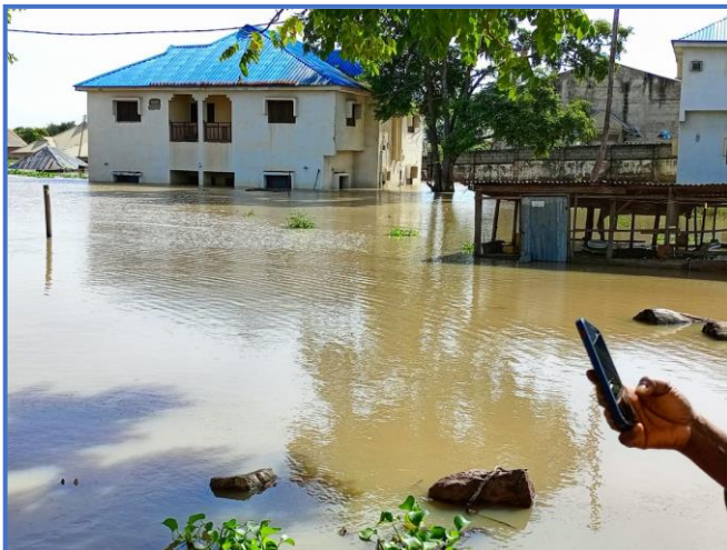
KONGONET Flood Impact Assessment team at Kogi State House of Assembly Quarters overtaken by flood.
